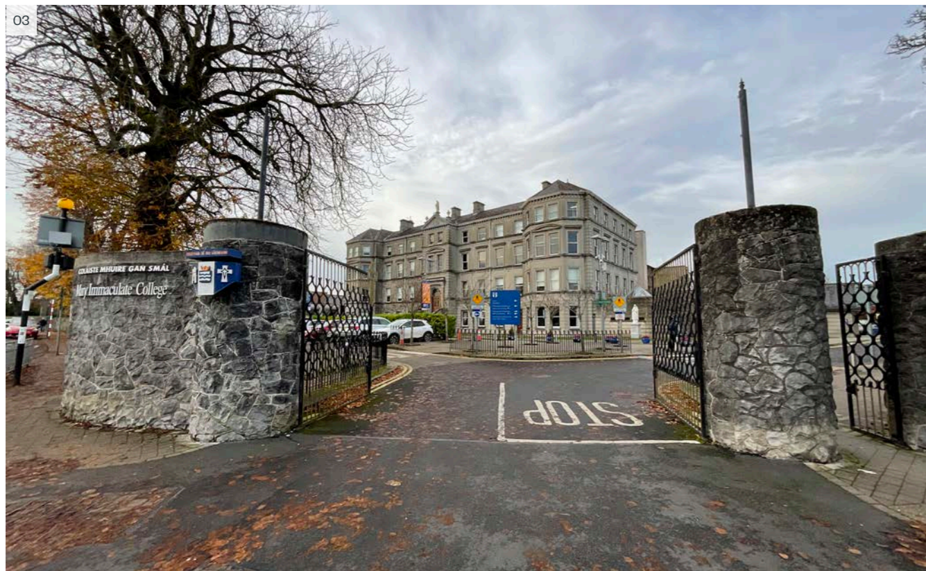
03 Vehicular access off South Circular Road with pinched pedestrian access gate
