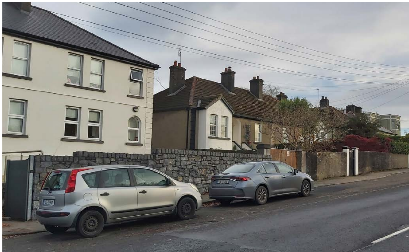
Ashbourne Avenue: Residential setting and scale of context (view facing east)
