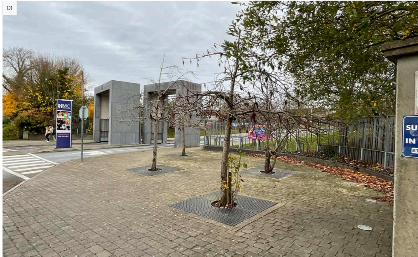
01 Main vehicular access is off Ashbourne Avenue, featuring striking access gateway elements
