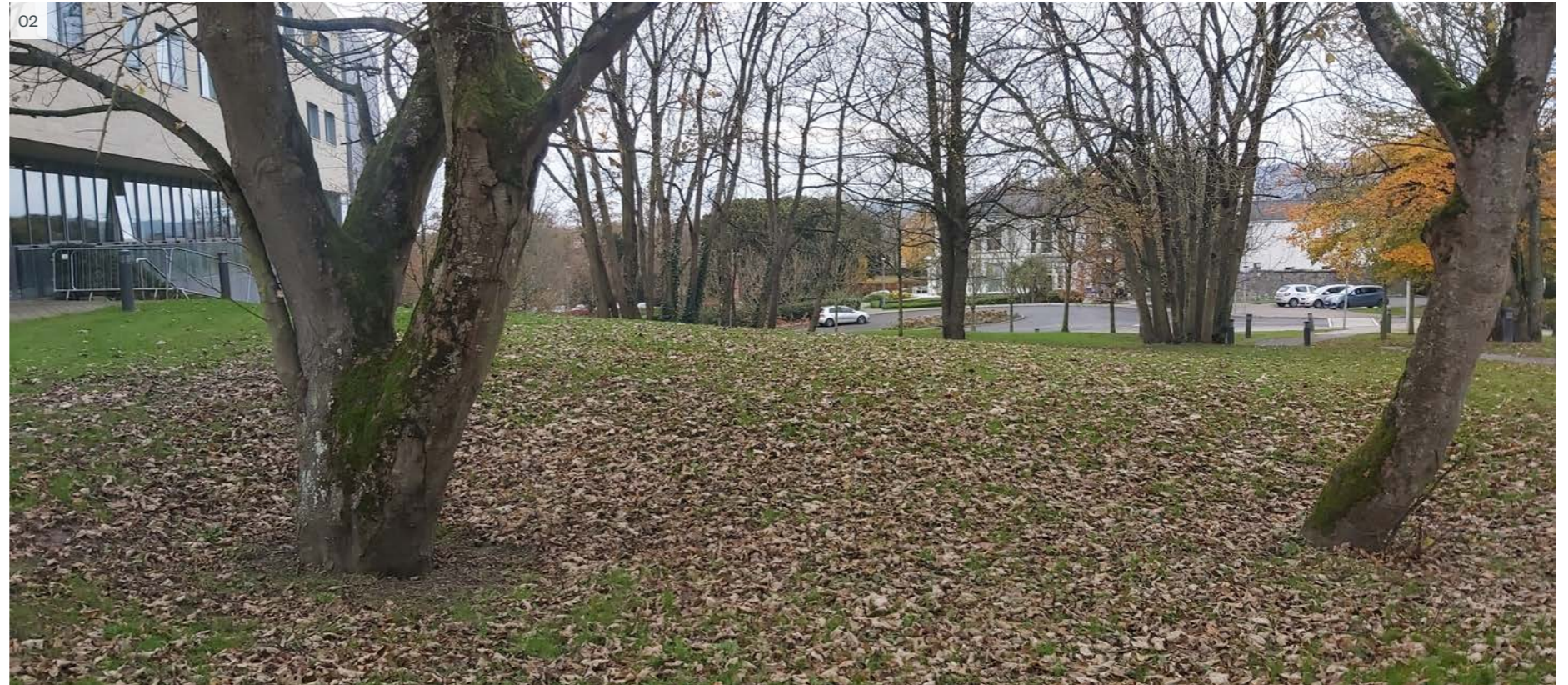
02 View west along sloping parkland topography towards the historic campus area - north-facing TARA Building elevation on the left with a long external staircase
