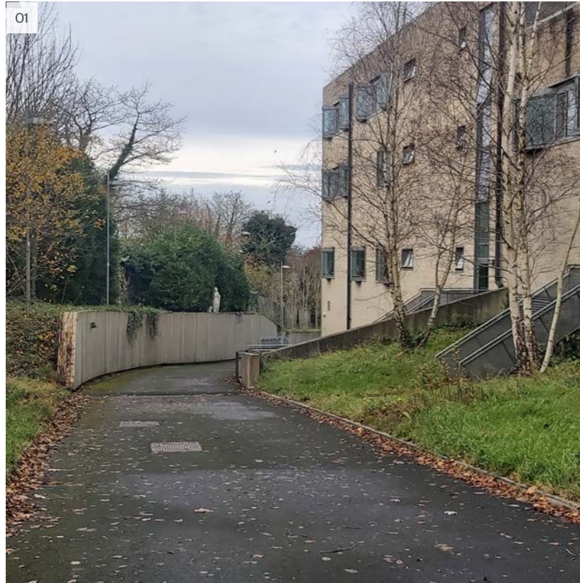
01 Sloping route (part 1:12) rear of TARA Building - primarily for service vehicles only
