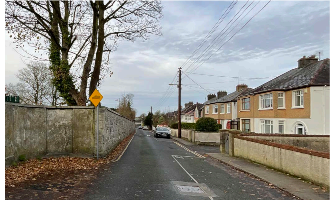
Summerville Avenue: Campus boundary wall fronting a residential setting (view facing west)
